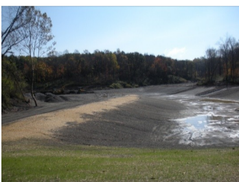
3-acre pond, completed mid-October
