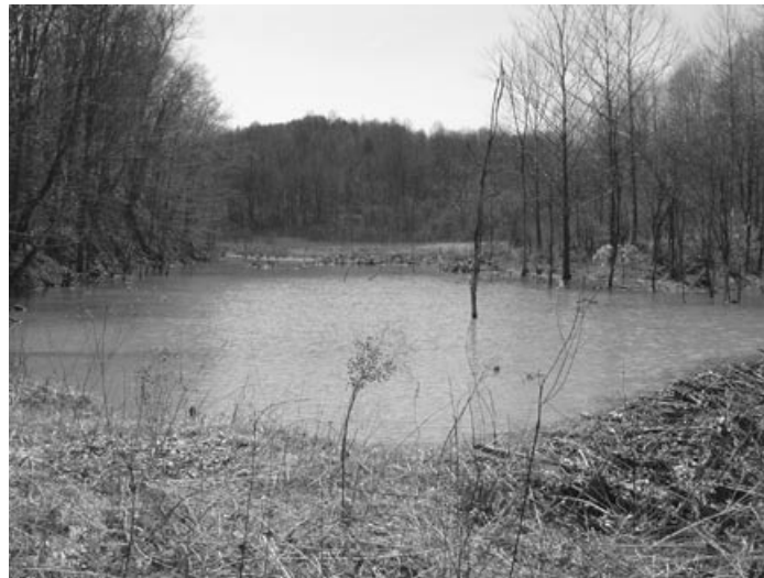
Water impounded by a beaver dam at Lost Run. A concrete dam will be constructed to increase the size of the pond, and a steel slag leach bed installed to neutralize acid mine drainage. Photo by Douglas Leed, ODNR
