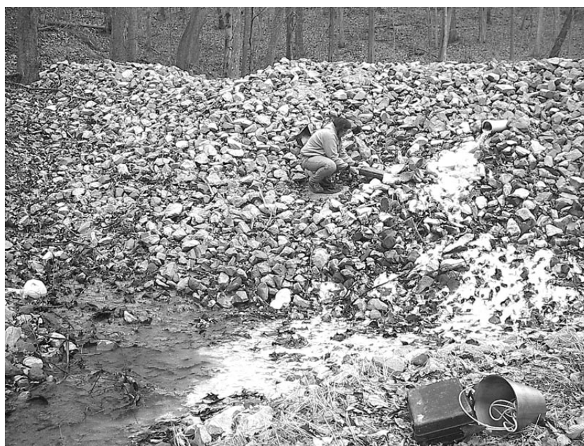
Water quality specialist Rebecca Black maintains an AMD treatment pond, which is causing thousands of pounds of iron (left) and aluminum (right) to fall out of solution as it improves the water's pH.
