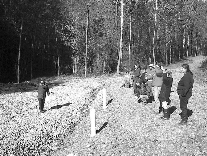
Mike shows how the new limestone leach bed will remove acid and metals from the water before it reaches the main creek.
