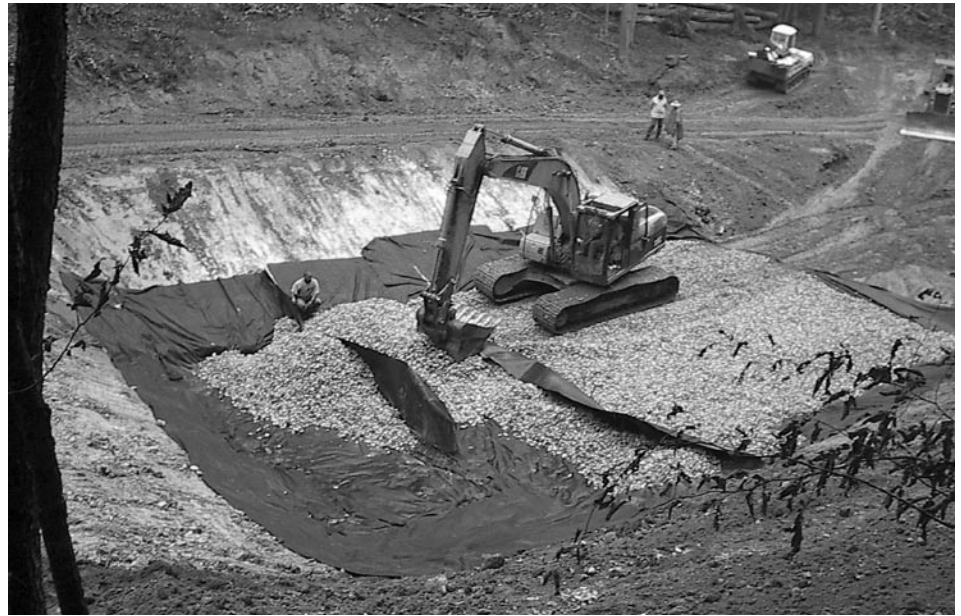
A crew from Tucson, Inc. places limestone rock into the impervious liner of a leachbed. Water flowing through the leachbed picks up alkalinity as it dissolves the limestone. Photo by Rebecca Black
