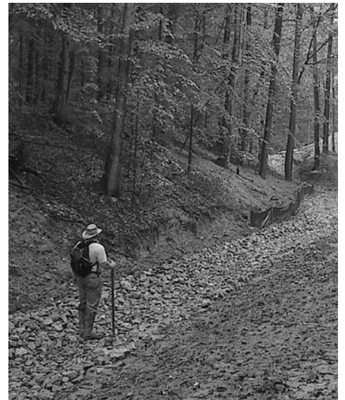
A crew from Tucson, Inc. places limestone rock into the impervious liner of a leachbed. Water flowing through the leachbed picks up alkalinity as it dissolves the limestone. Photo by Rebecca Black
