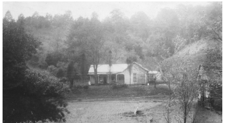
Top: Bucyrus Erie B2 steam shovel on location in Sand Run. Below: The Kings' house in Sand Run. Family photos courtesy of Kathryn King Gardner Weber.
