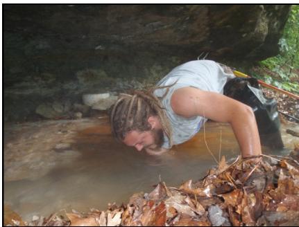
Above: Nate Schlater cleaning out the inflow pipe to Essex Doser
